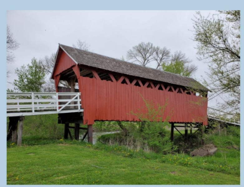
The timber for the bridge was cottonwood, a native lumber from donated trees that were cut to size by a local saw mill. Over 20 years the wood had shrunk, warped and sagged to the point where the safety of the bridge was of serious concern. The slow, but unrelenting movement caused the whole structure to twist in a way that put new stresses and loads on beams that were not intended to support.
