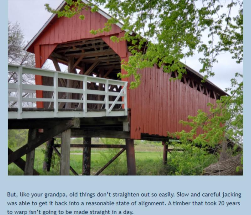
the bridge. But that would have ruined its charming exterior so the team worked to weave new posts and knee braces through the existing structure on the inside of the bridge. This required some very careful coordination with the contractor as they threaded the new struts through the old without taking the old apart.
