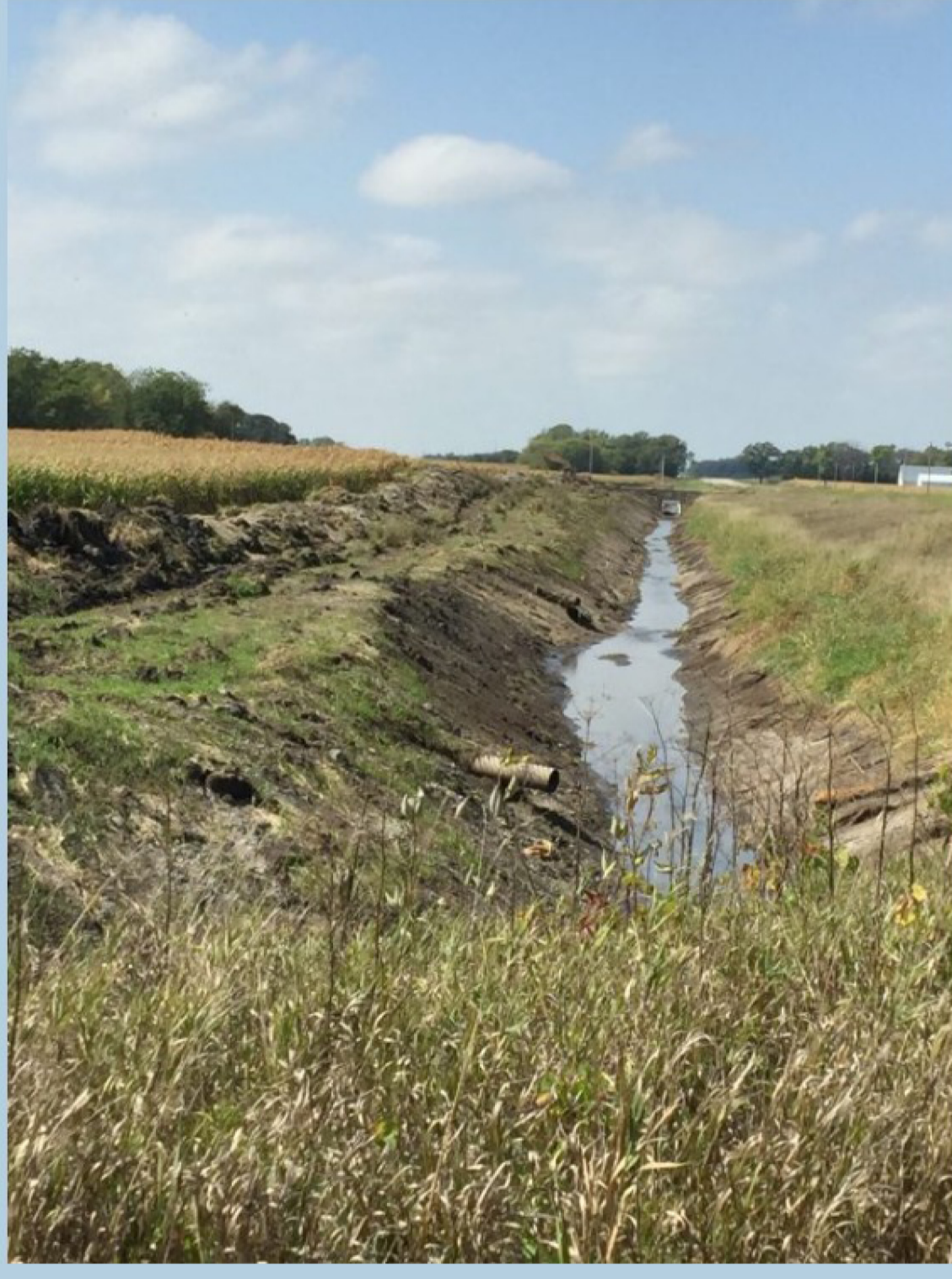
Recently cleaned out drainage ditch and new concrete box culvert in the background. Unleveled spoil bank on the left was leveled after material dried significantly.
