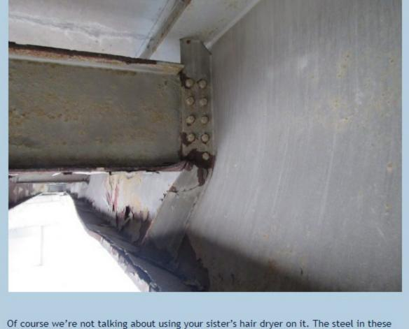
girders is an inch and more in thickness and it takes some serious heat to make a difference. But isn't just simply a matter of aiming a blast furnace at it. The temperature of the steel must be kept within a very specific range or its internal properties will change, and it will lose its strength or become too brittle.
