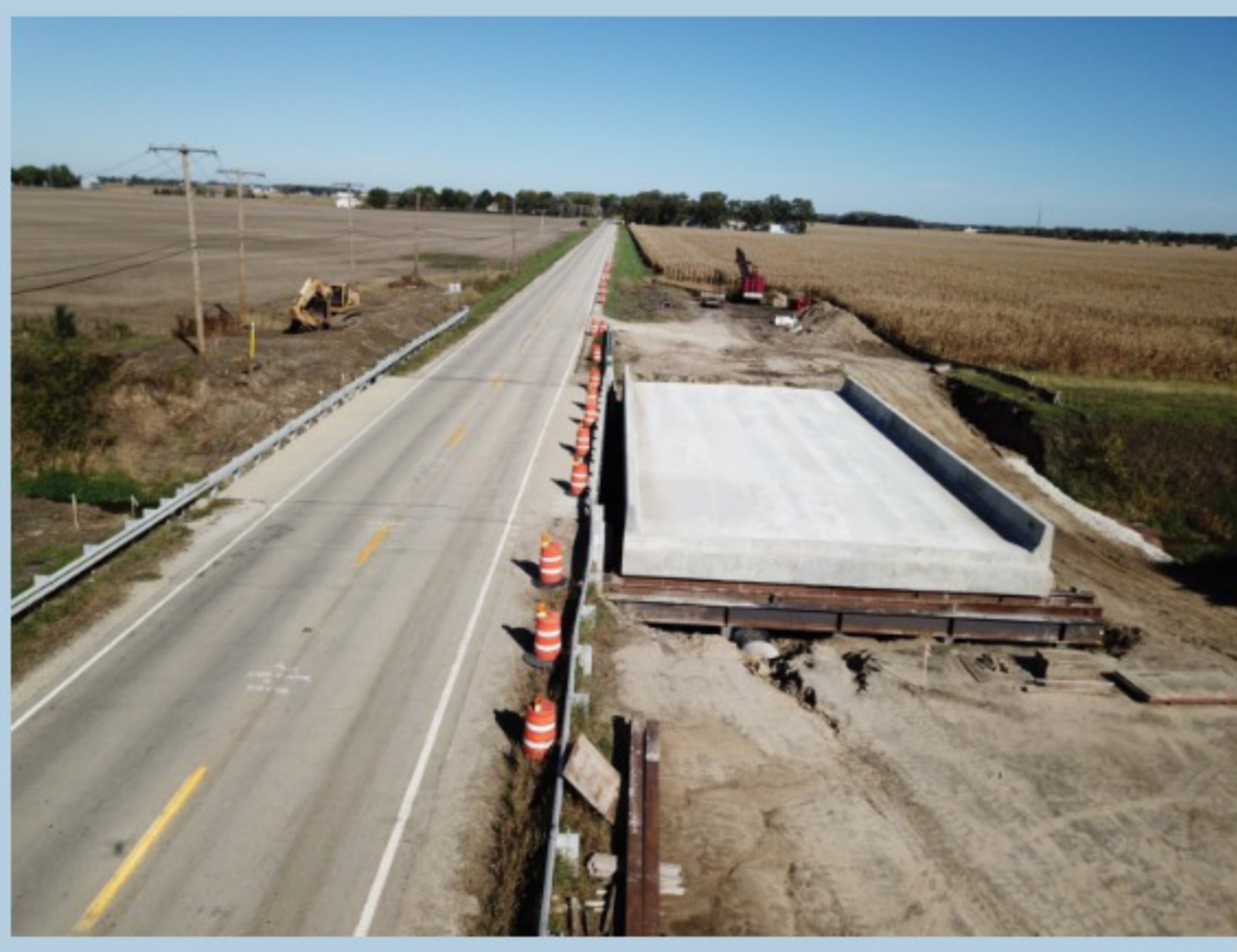
Aerial Image of Superstructure Constructed on Temporary Bents
