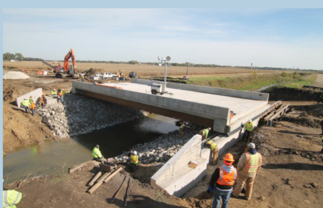
Lateral slide in progress
