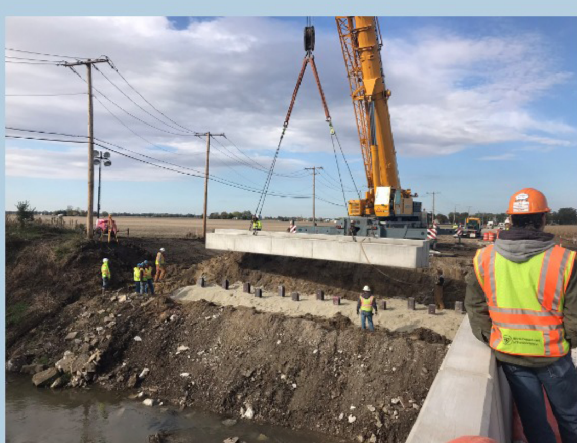
Precast abutment cap being installed
