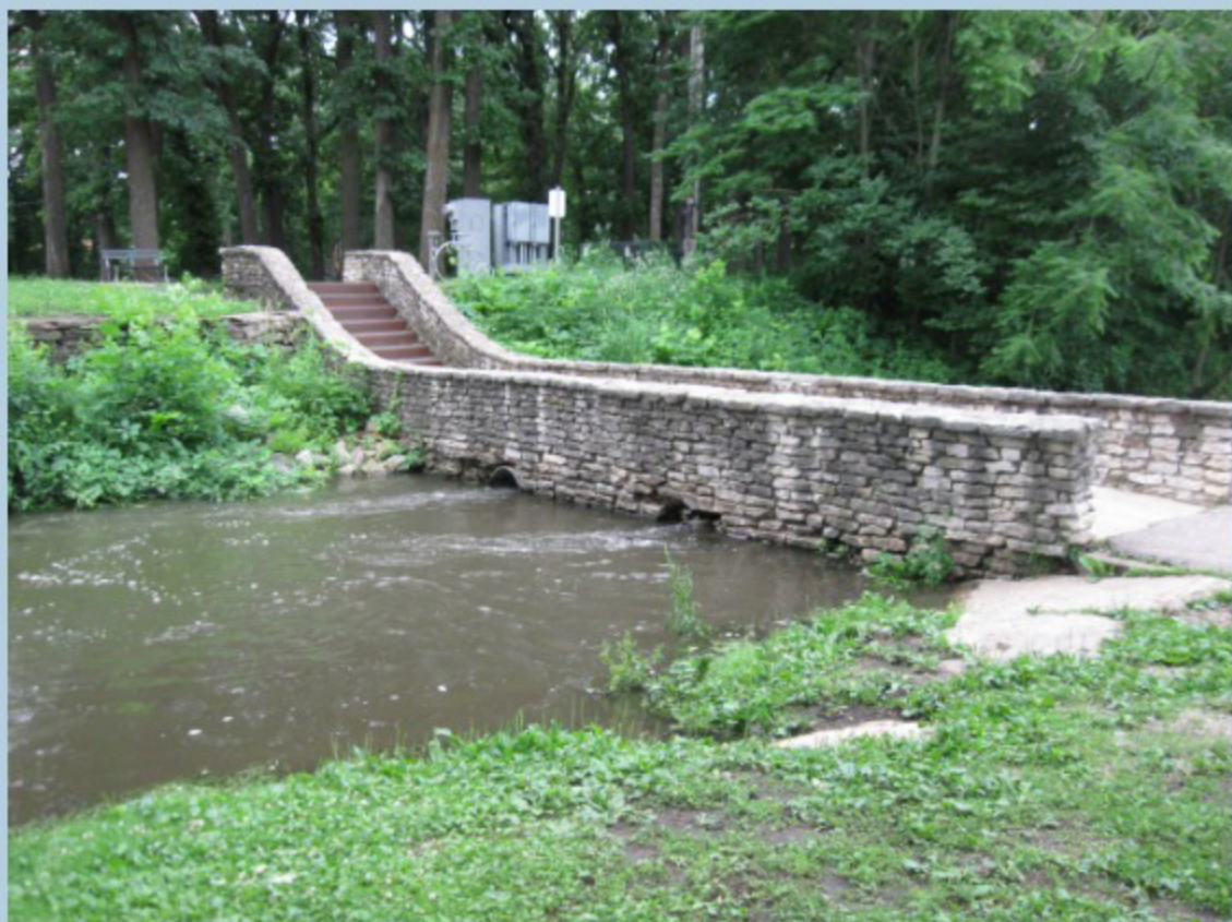
Stone Bridge Before
