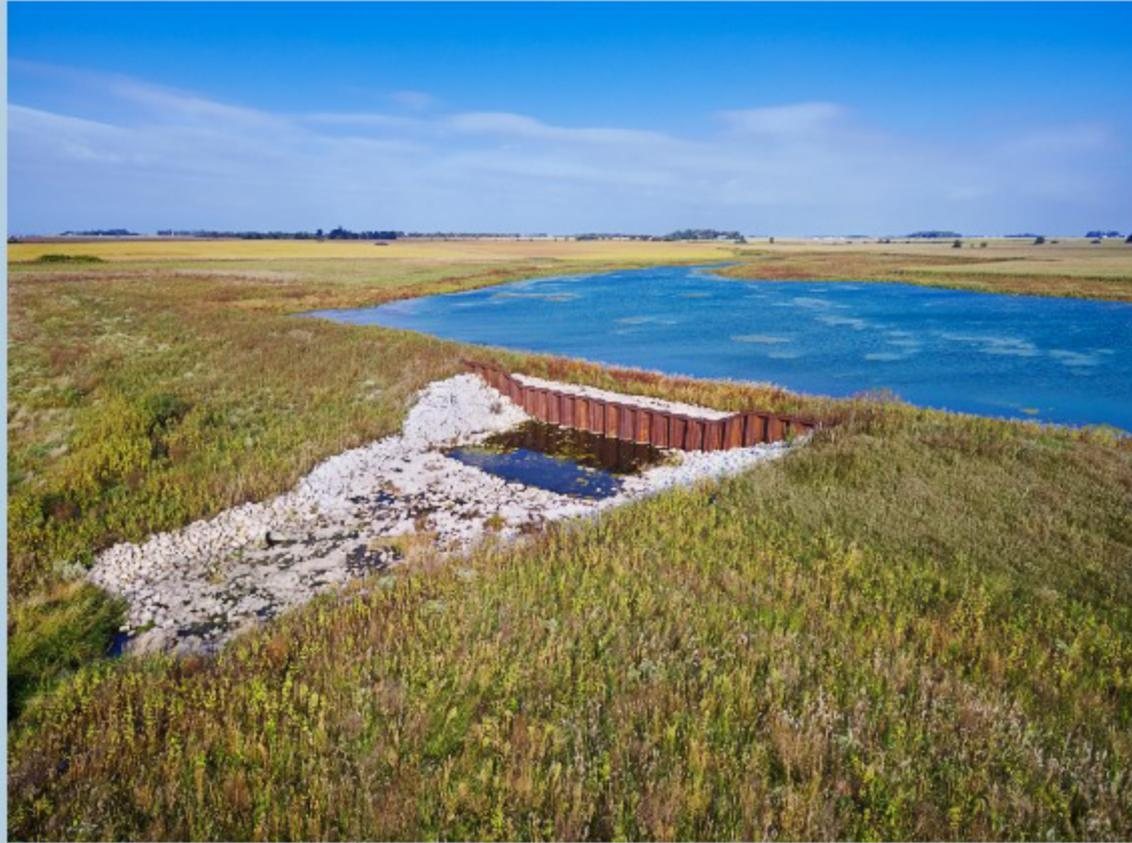
Most often a CREP project will involve the construction of a low dam in order to flood a large area to a depth of less than three feet. Engineering design includes a study of the hydraulics, a geotechnical analysis of the underlying soil and the design of the dam structure, often constructed from sheet pile weirs. Since, over decades, much of the drainage has been put into buried tiles, these drain lines have to be located and then diverted to discharge into the new wetland area.
