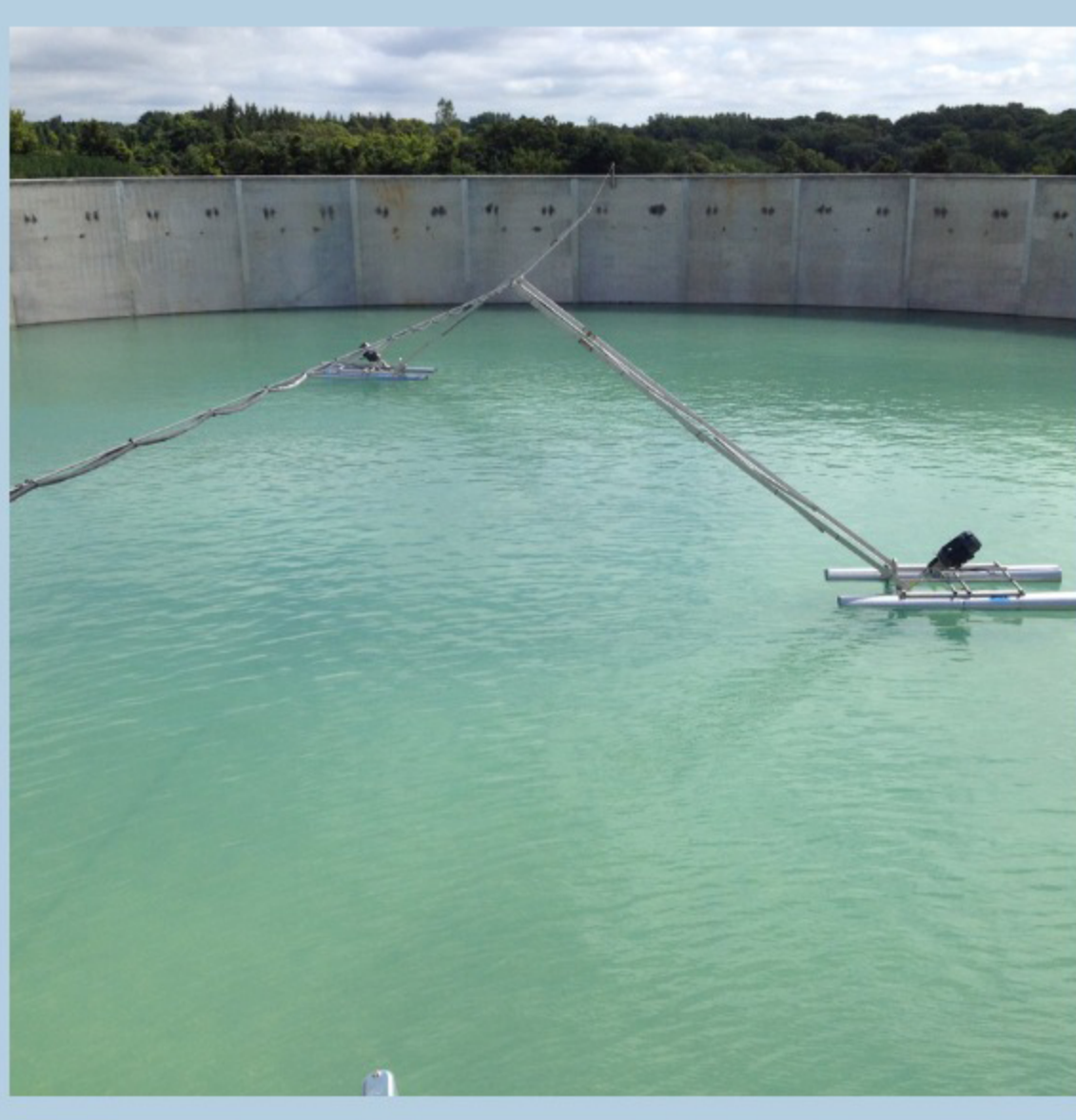
Clean Water Test of the Aeration Mixer Tank
