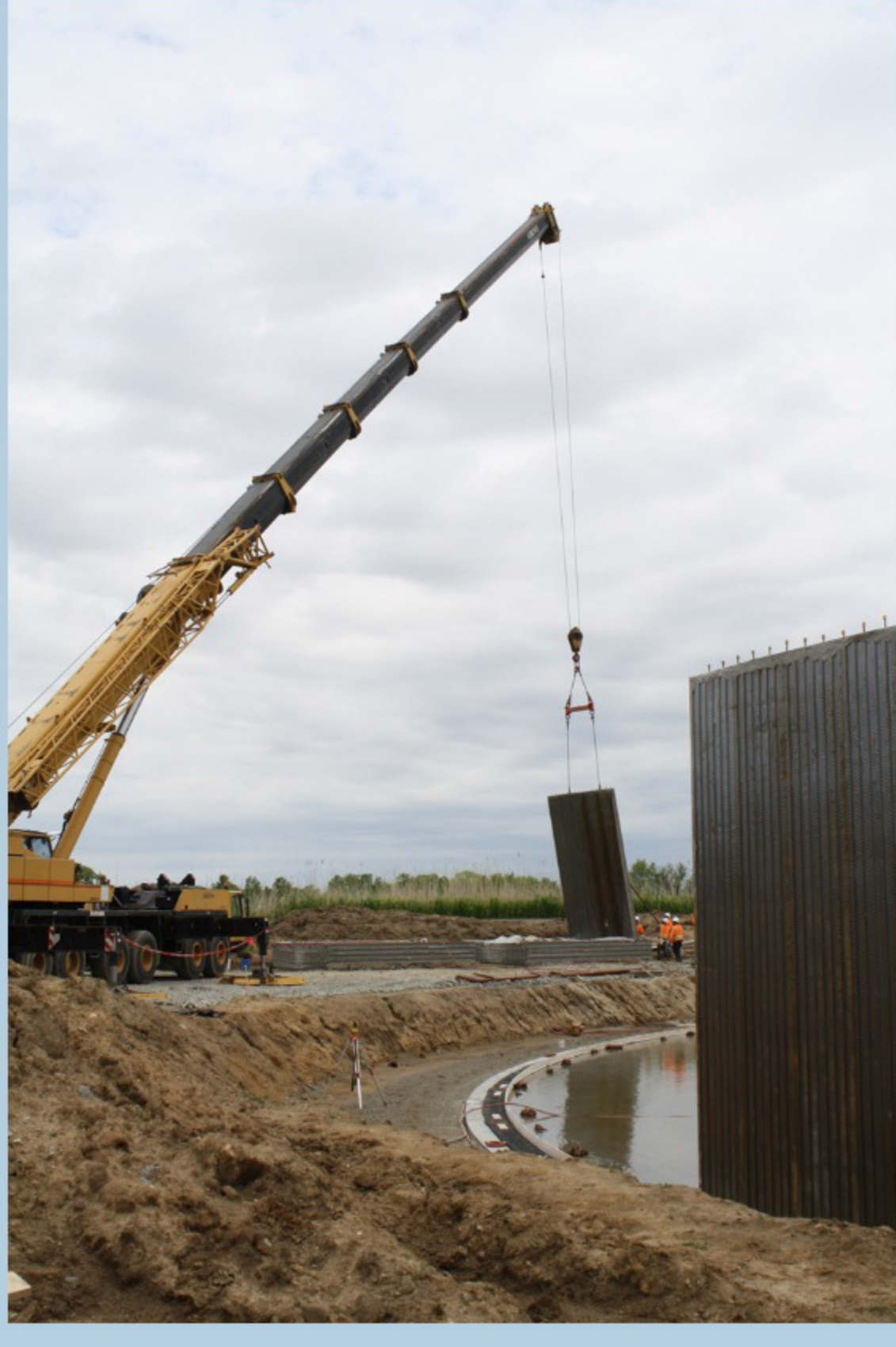
Panel Erection
