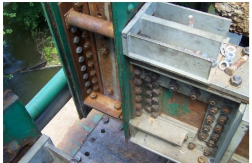
*Floorbeam and truss strengthening system*
