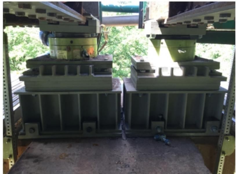
*Jacking system under the end floorbeams*
