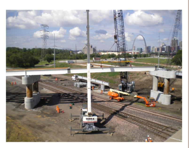
The new MLK Connector over Illinois Rte. 3 in St. Clair County is an eight-span, continuous horizontally curved composite steel girder bridge that crosses an active roadway and two railway tracks. In other words, it's complex. So the Department of Transportation required that a Structural Engineer prepare a steel erection plan prior to construction to consider and account for the stresses imposed through the construction period.
