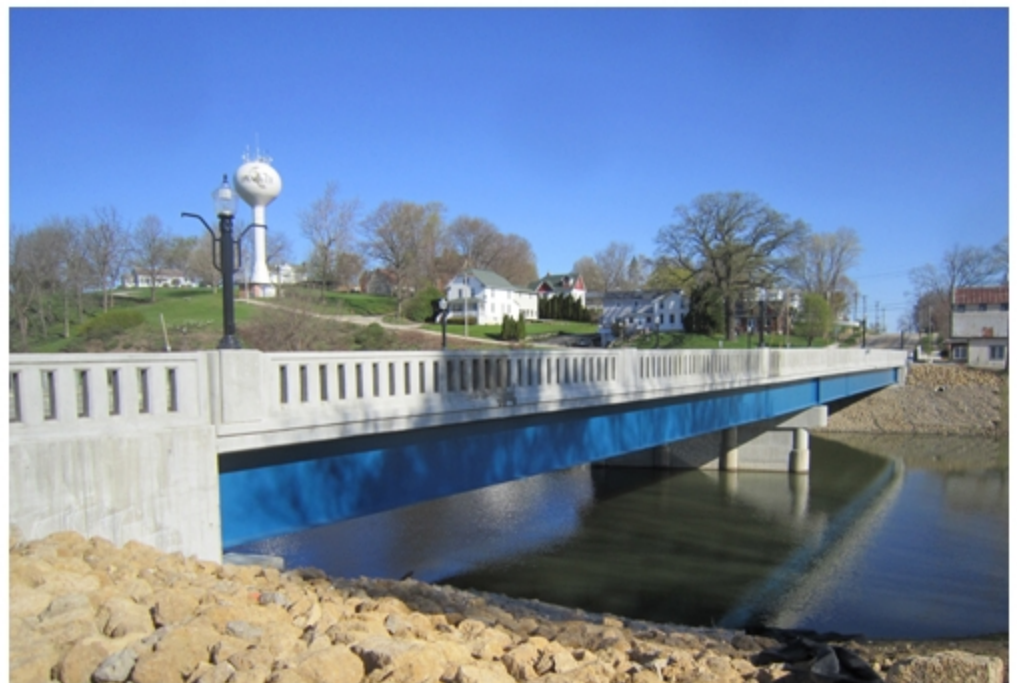
IL 84 Bridge After Construction
