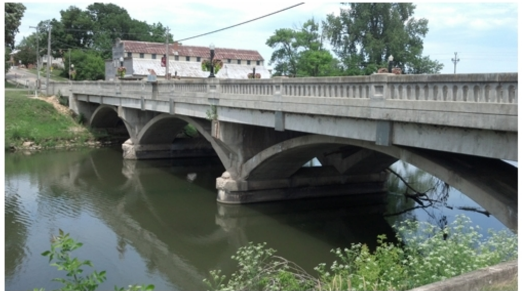
IL 84 Bridge Prior to Construction
