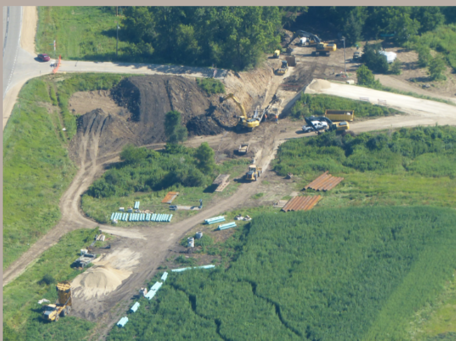
Utilities at Olde Davenport Road under construction
