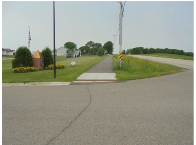
Before and after photos for Byron, Minnesota Safe Routes to School project
