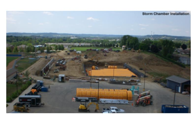
As designers worked to determine how to control stormwater runoff, they realized that, about 150 feet west and many feet underground from the new facility, lay an old abandoned lead mine shaft. If stormwater was to find its way into the old mine, erosion, sinkholes and lead contamination could easily result.
