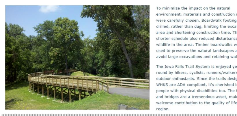
To minimize the impact on the natural environment, materials and construction methods were carefully chosen. Boardwalk footings were drilled, rather than dug, limiting the excavation area and shortening construction time. The shorter schedule also reduced disturbances to wildlife in the area. Timber boardwalks were used to preserve the natural landscapes and avoid large excavations and retaining walls.
